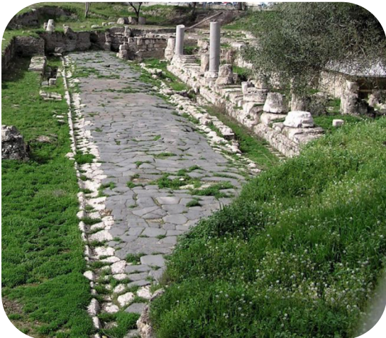
First century BC Roman road in Tarsus . The pavement is made of black basalt with gutters of white limestone.
